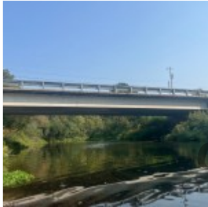
County Road N Bridge
