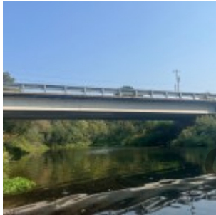
County Road N Bridge
