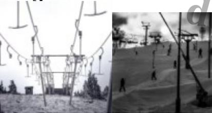
A drag lift is similar to a tow rope but has a bar hanging from a cable.
